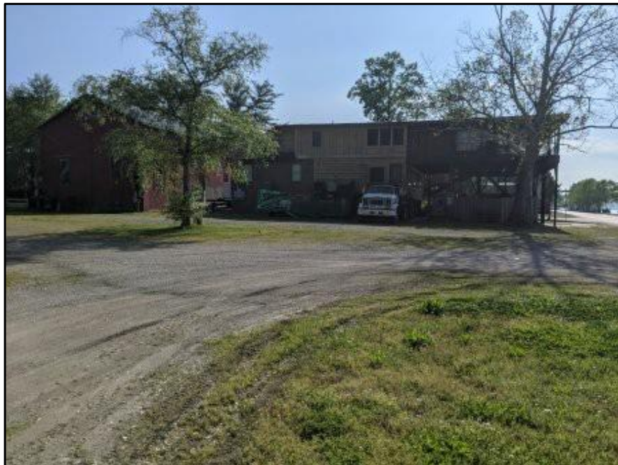
8: View of the east adjoining vacant property and residential beyond.
