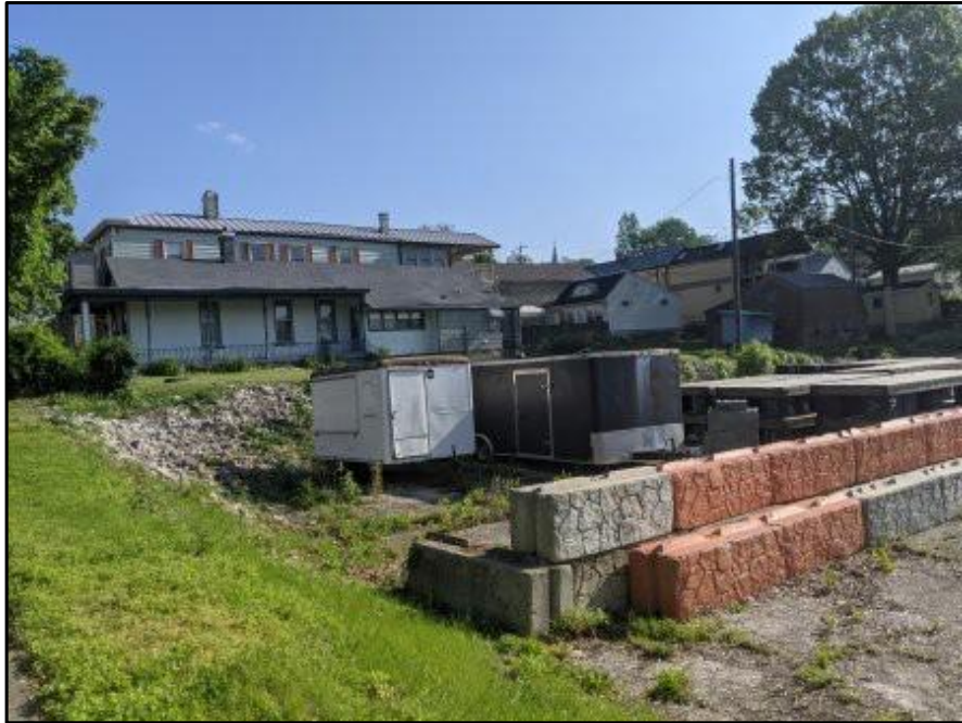
5: View of the north adjoining residential property.
