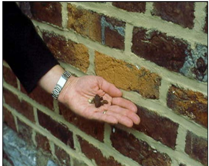
NO-Abrasive cleaning and repointing with inappropriate mortar removes the exterior "crust" and can lead to deterioration (above) and spalling (below).
