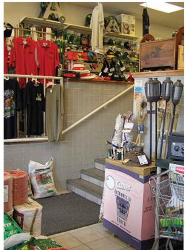
After entering the business, shoppers can either use an ADA compliant ramp (left) or go up the stairs to the new first floor level (right). The entrance area has been retrofitted with flood resistant materials including a tile floor and tile surfaces on the stairs.
