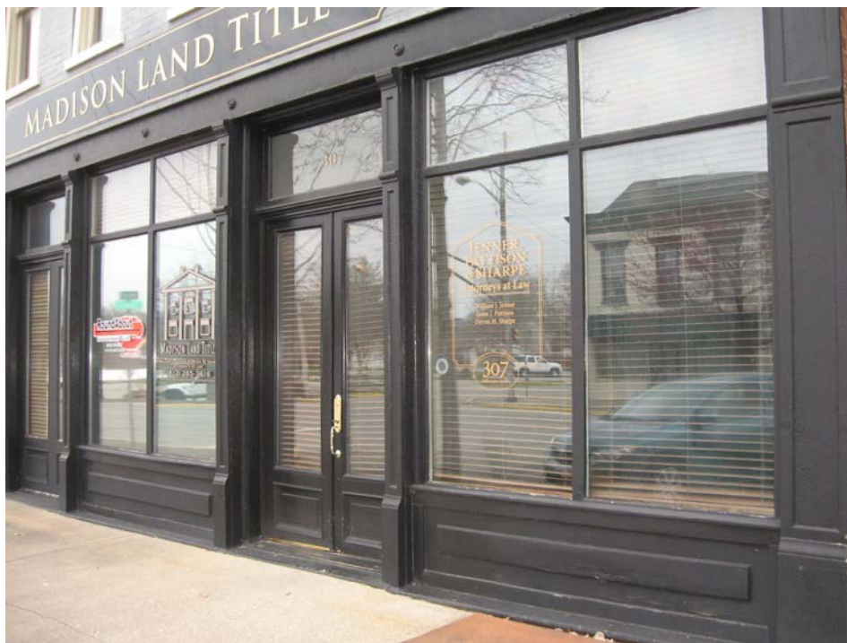
Examples of appropriately rebuilt storefronts are at 214 E. Main Street (above) and 307 Jefferson Street (below). They have display windows on paneled frame bulkheads, paneled and single-light doors other traditional features.
