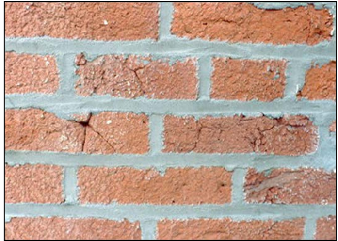
NO-Abrasive cleaning and repointing with inappropriate mortar removes the exterior "crust" and can lead to deterioration (above) and spalling (below).
