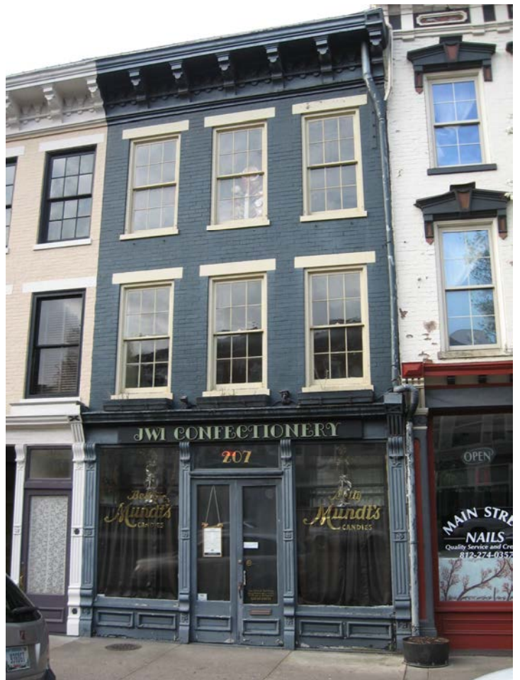
Two-Part commercial block building at 207 W. Main Street. The building retains much of its cast iron storefront and upper façade of sheet metal hood molding over the windows and cornice at the roofline.
