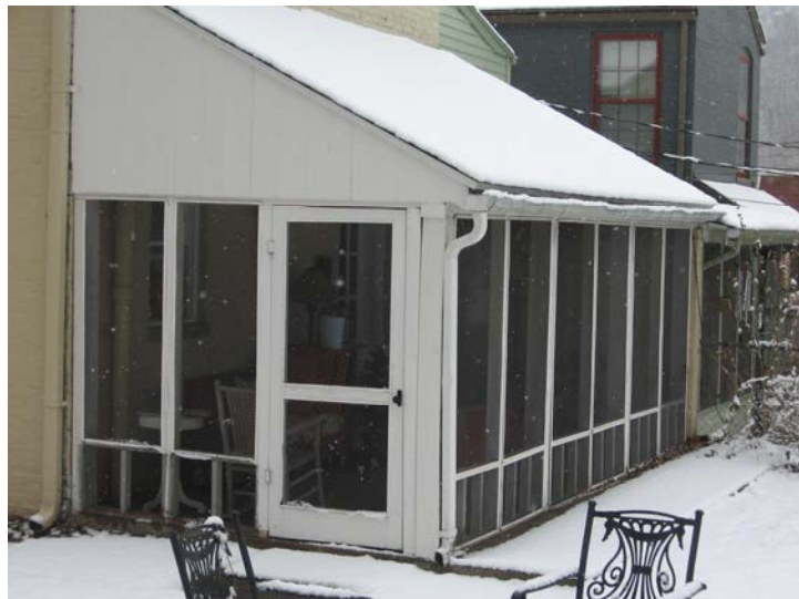
YES-Porches should be screened with as limited structural framing as possible (516 West Street, above, and 107 E. Third Street, below).
