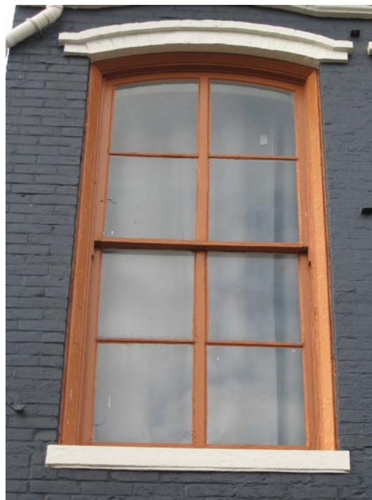
Four-over-four wood sash, 315 W. Main Street.
