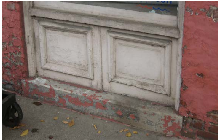
Preserve and maintain original frame bulkheads as at 110 W. Main Street (above) and 221 E. Main Street (below).
