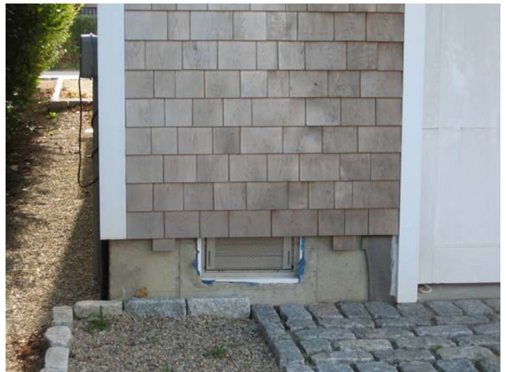
FEMA standard flood vents can be retrofitted into historic brick foundations (above) and poured concrete foundations (below).
