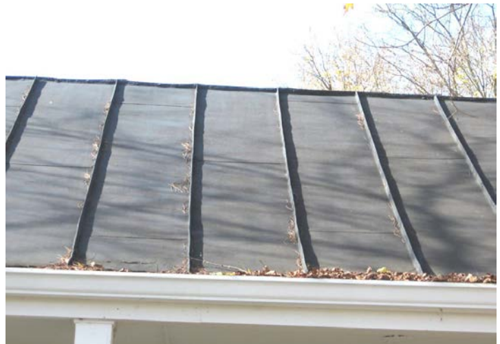
Metal standing-seam roofs from the nineteenth and early twentieth centuries should be preserved and maintained (902 W. First Street).
