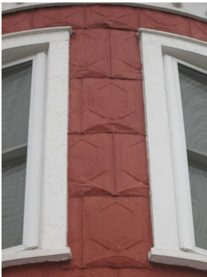
Sheet metal stamped into various patterns was also used as an exterior wall surface. At left is a hexagonal design in the upper façade at 301 Walnut Street. At right is sheet metal designed to look like stone at 322 Mulberry Street.
