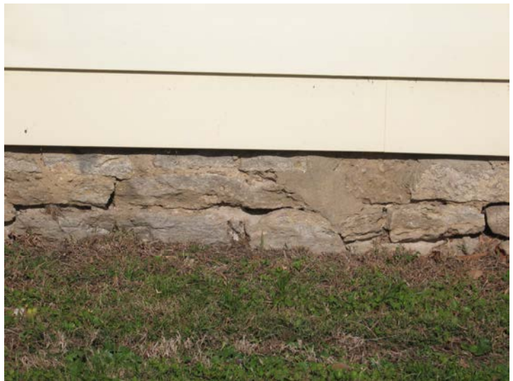
Stone foundation at 1002 W. Second Street.
