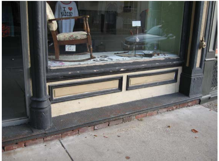
Preserve and maintain original frame bulkheads as at 110 W. Main Street (above) and 221 E. Main Street (below).
