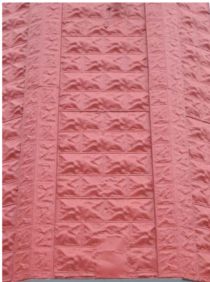
Sheet metal stamped into various patterns was also used as an exterior wall surface. At left is a hexagonal design in the upper façade at 301 Walnut Street. At right is sheet metal designed to look like stone at 322 Mulberry Street.
