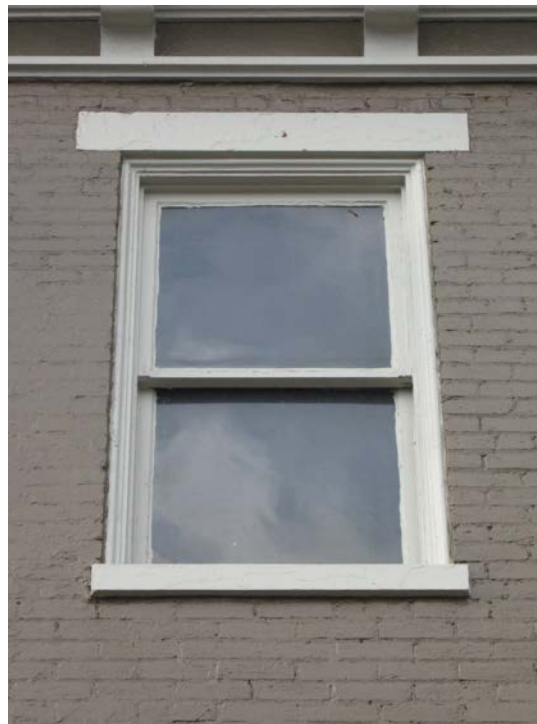
One-over-one wood sash, 329 W. Main Street.
