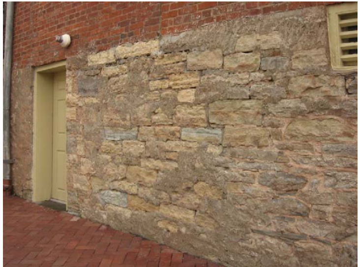
Stone foundation at 217 W. Second Street.
