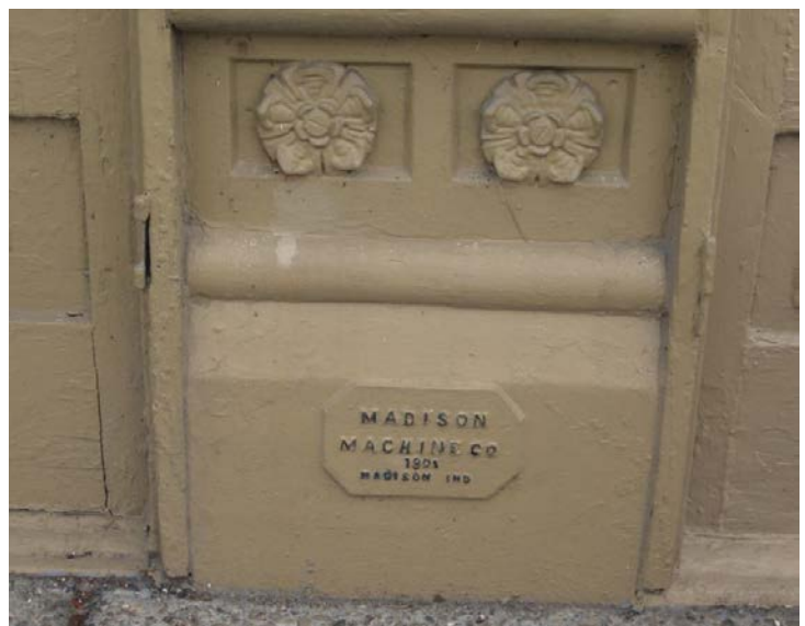
The cast iron pilaster at 629 W. Main Street was manufactured by the Madison Machine Company in 1901.
