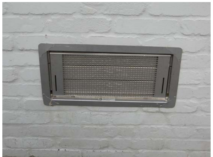
FEMA standard flood vents can be retrofitted into historic brick foundations (above) and poured concrete foundations (below).
