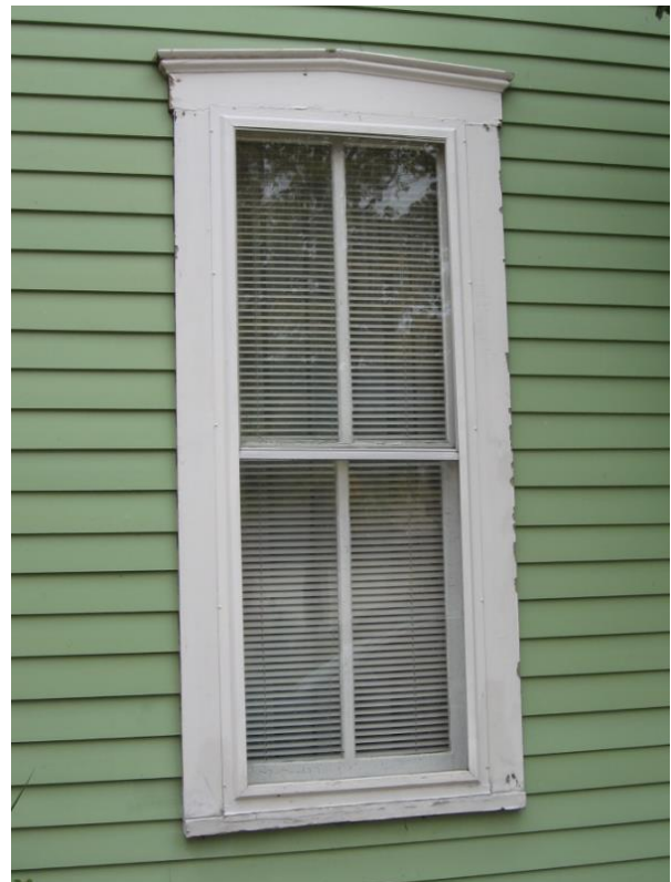
By the mid-nineteenth century, two-over-two sash windows were common (410 Broadway Street).
