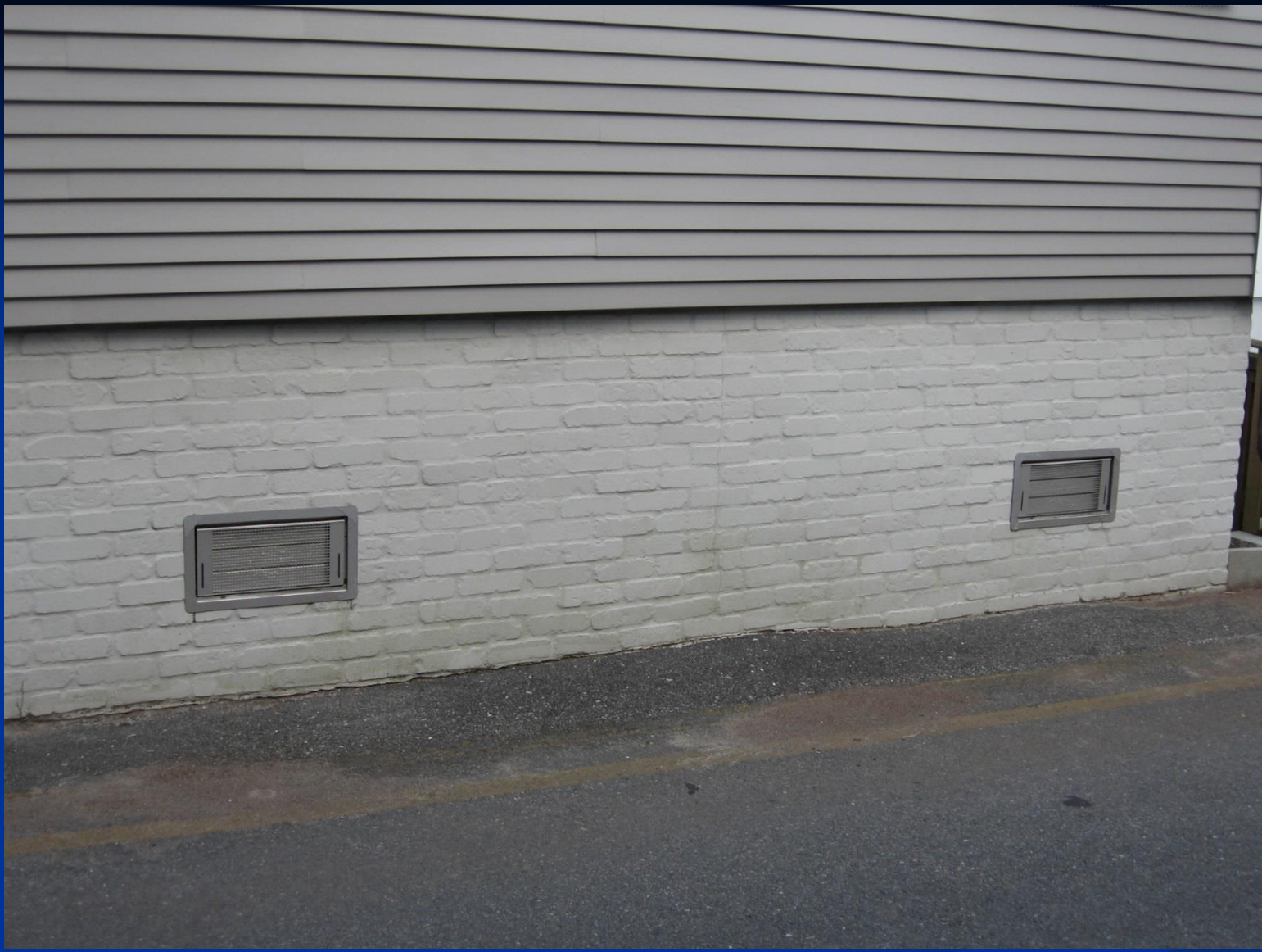
Flood Vents Added to a Brick Foundation
