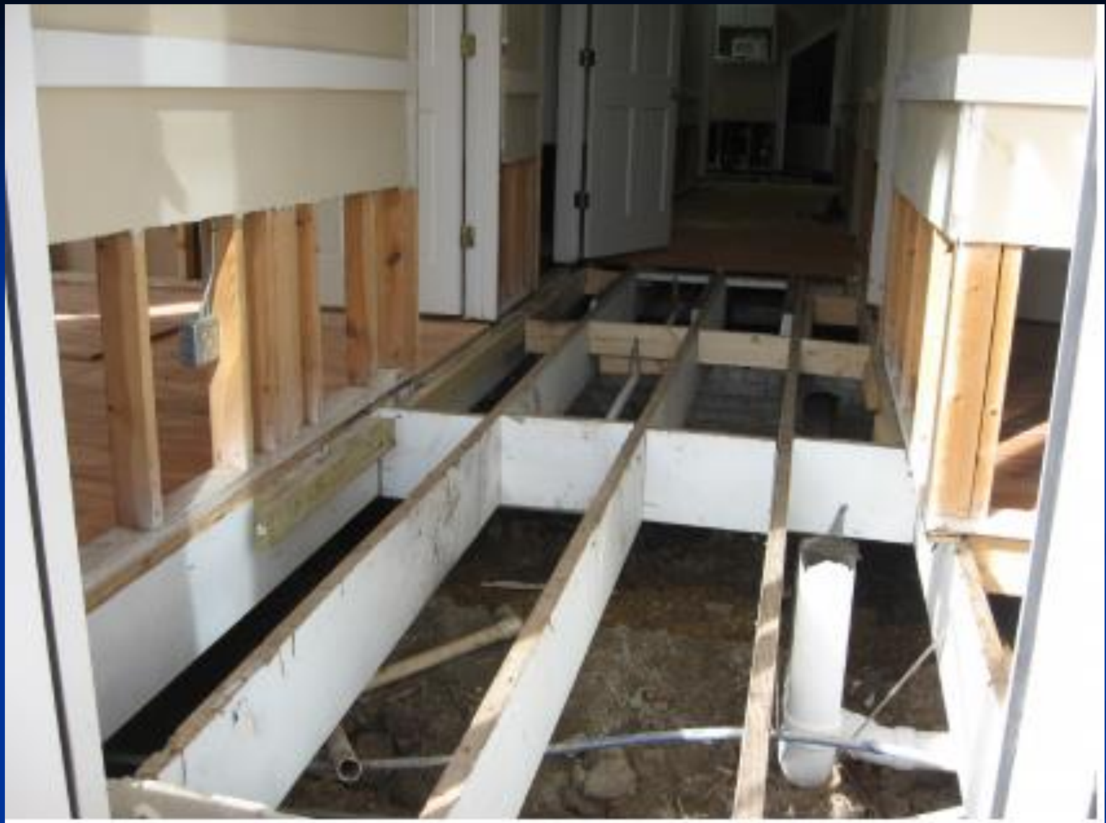
Wet Flood Proofing – Retrofit with Water-Resistant Materials
