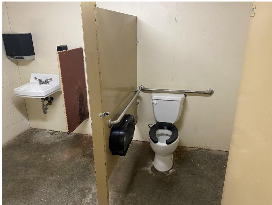
Rucker Sports Complex South Men's Restroom
