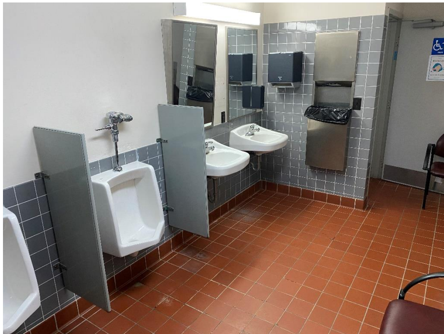
Sunrise Golf Course Men's Restroom
