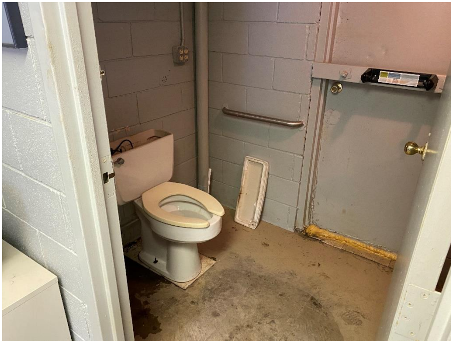
Regatta Office Restroom
