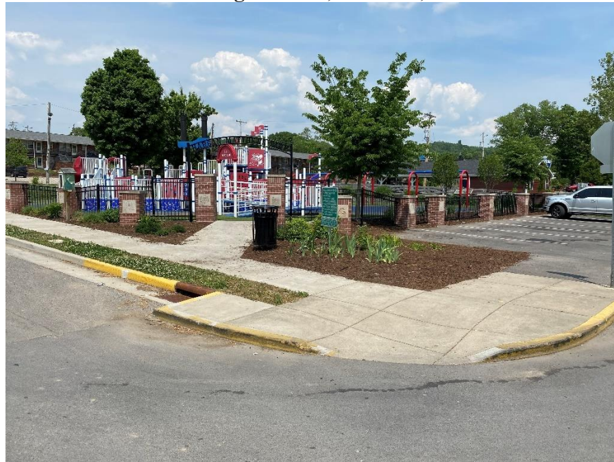
Hargan-Matthews Entrance and Parking Area
