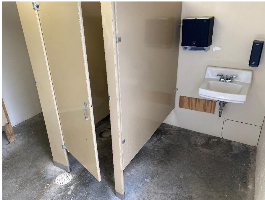
Rucker Sports Complex South Women's Restroom
