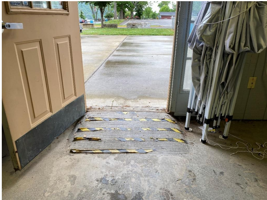
Regatta Office Entryway Ramp
