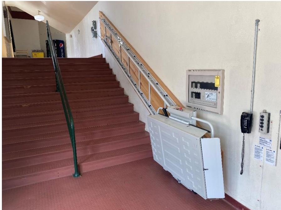
Brown Gymnasium Stairs and Chair Lift
