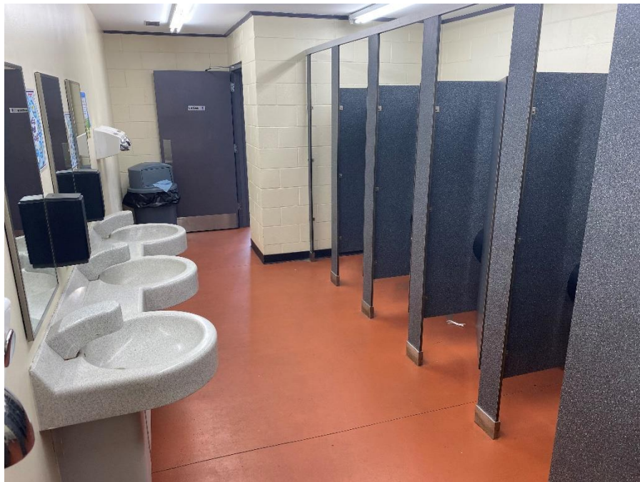
Comfort Station Women's Restroom
