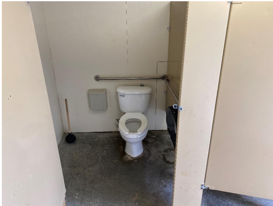
Rucker Sports Complex South Women's Restroom
