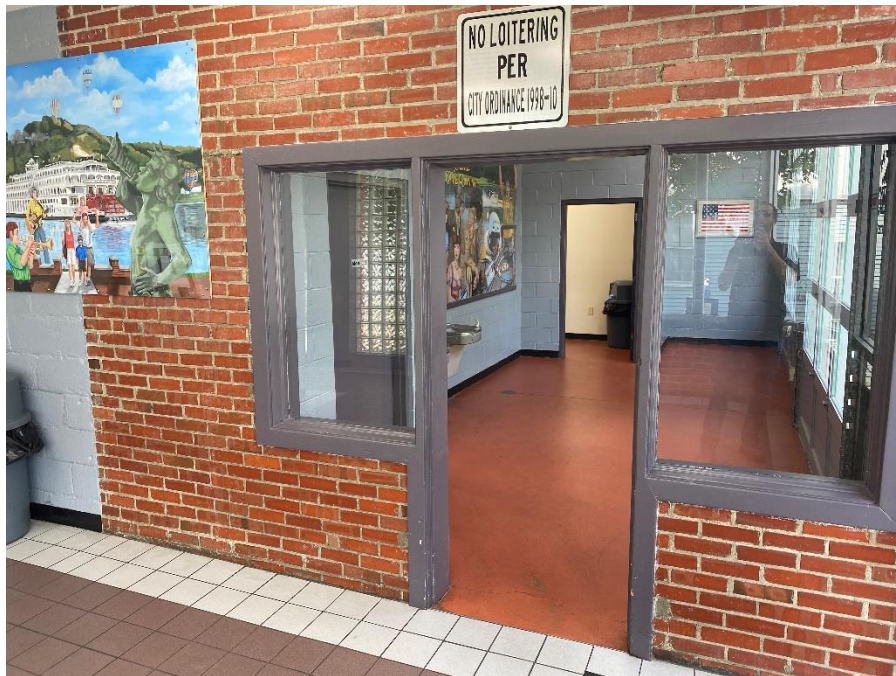
Comfort Station Hallway
