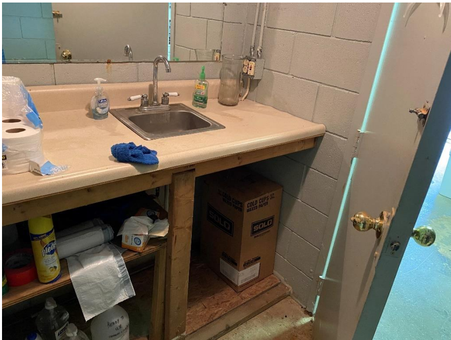
Regatta Office Restroom
