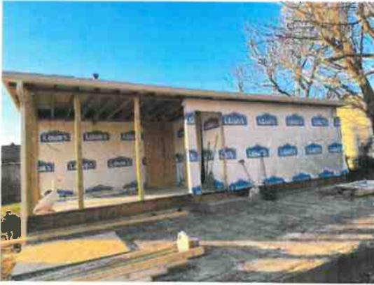
Line 2, 3, 15 framing, wrapped, **prepped** for siding
