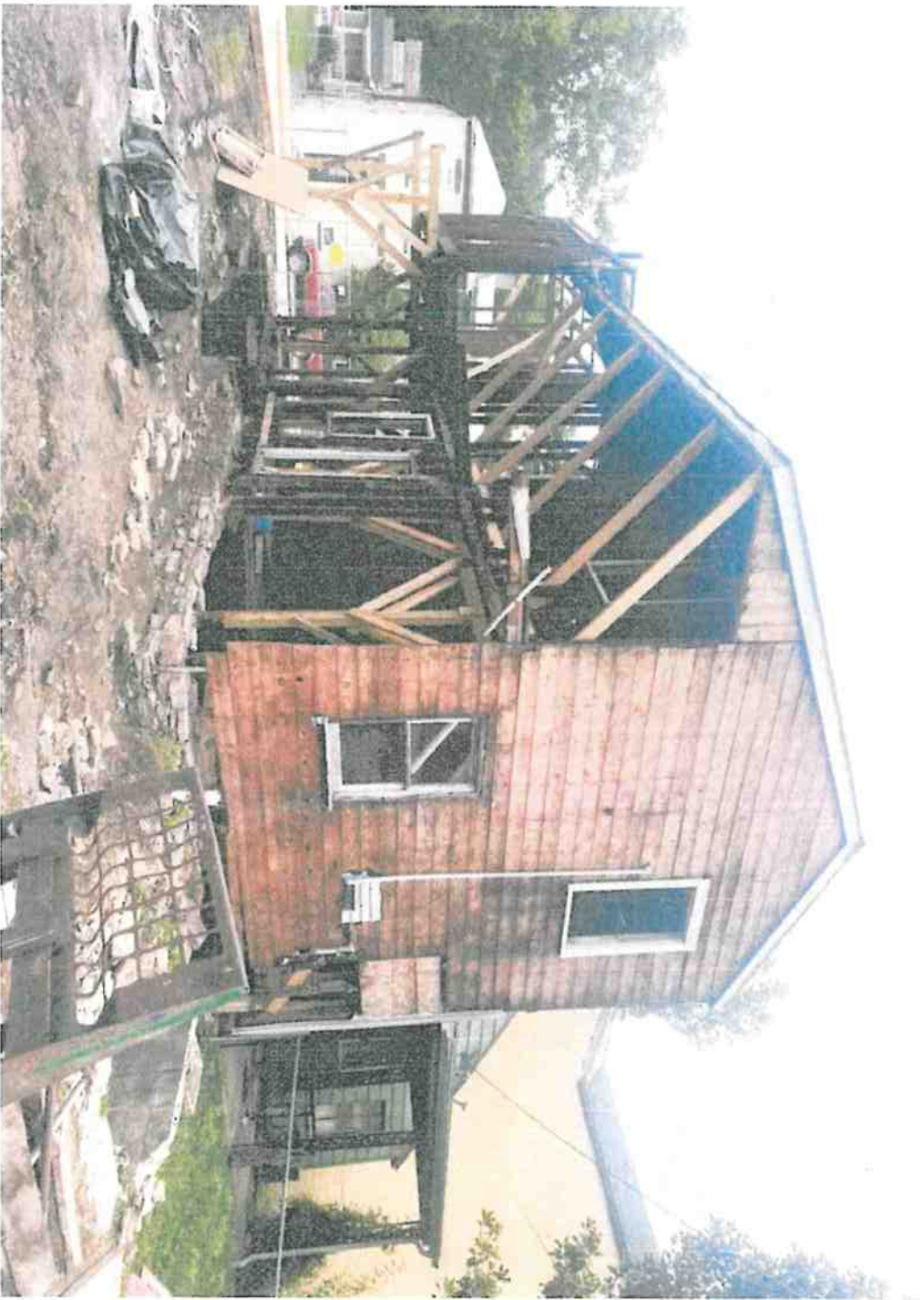
Demo and temporary support of the original structure
