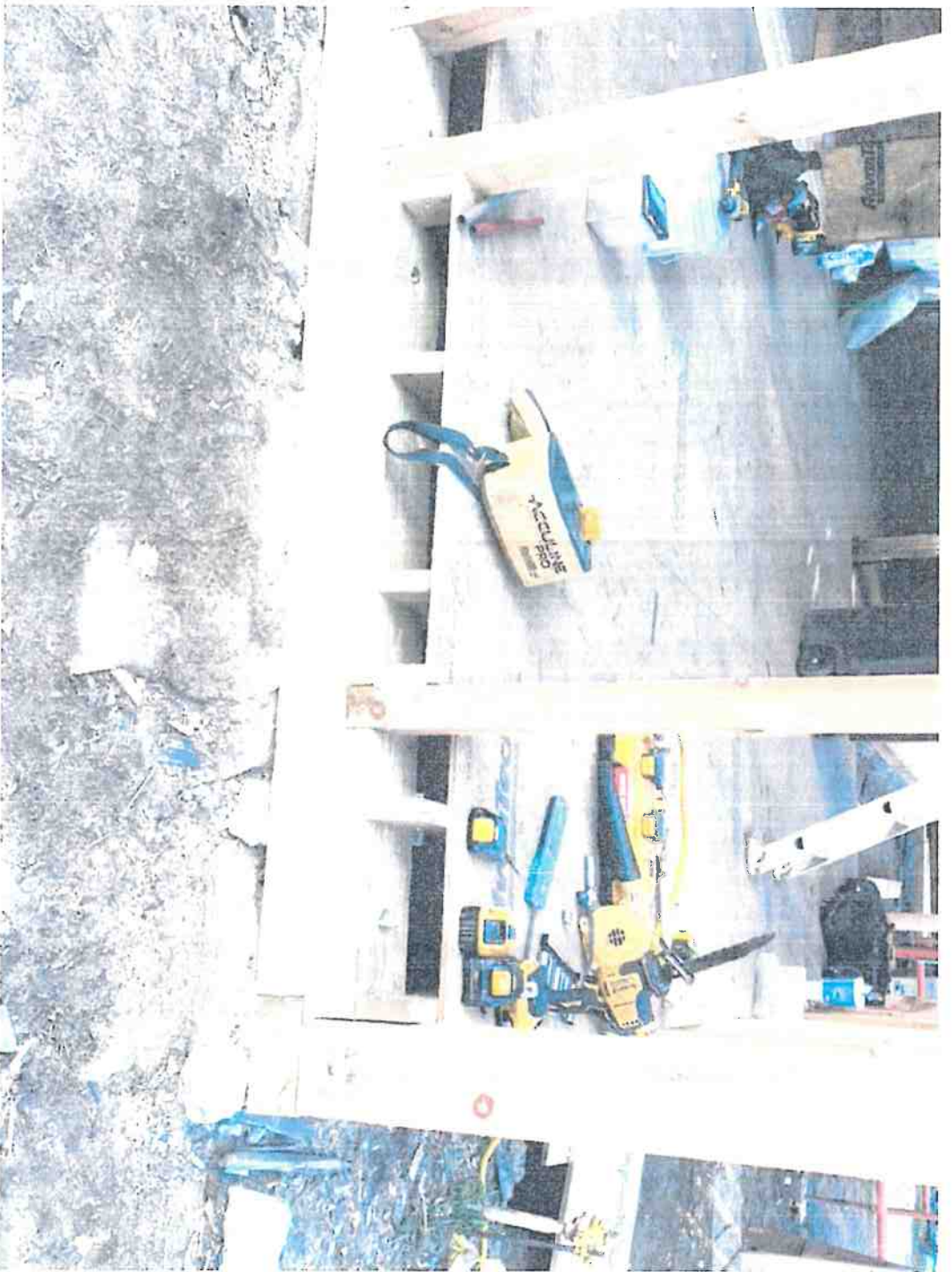
New sill beams and mortised wall framing
