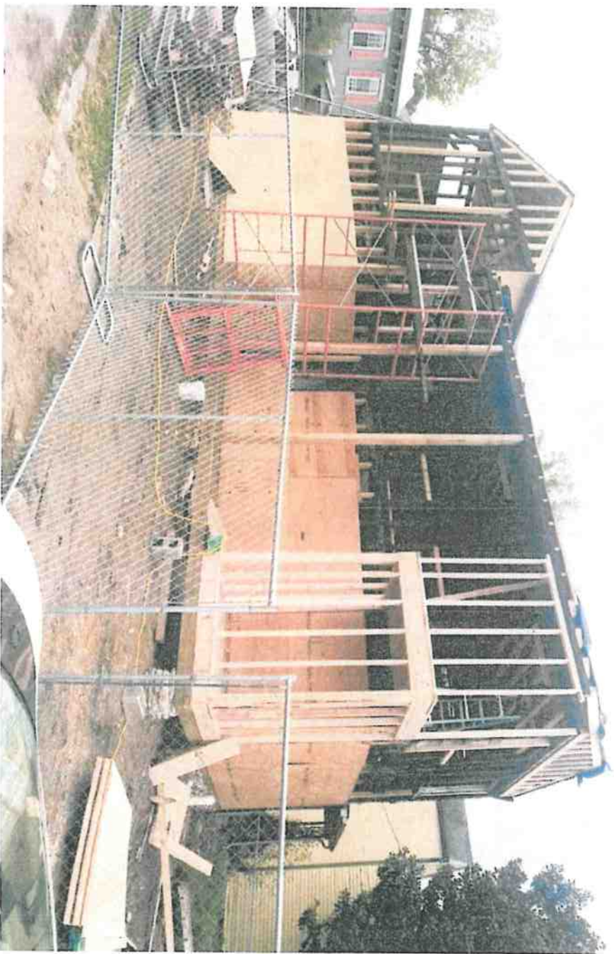
Reframed 1845 shell. Beginning plywood bracing
