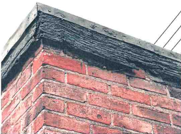
Rotted fascia boards on both buildings
