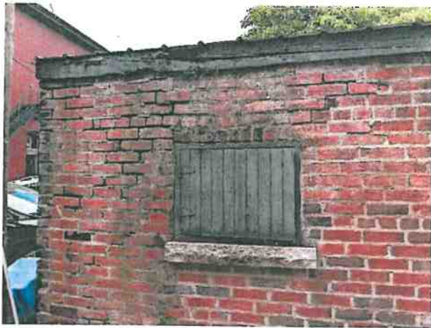
Window cover doesn't close on Donkey barn, rotted fascia board, and brick work needed
