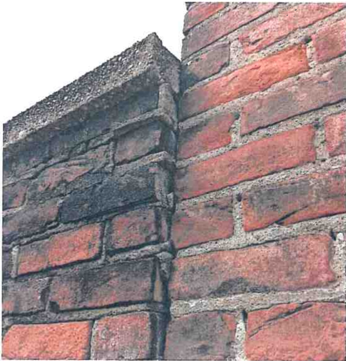
Evidence of leaning wall along alley
