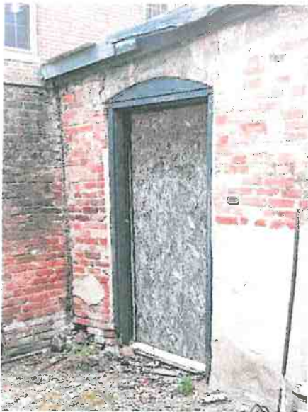
Door missing Southeast corner of Donkey Barn, more evidence of rotted fascia board
