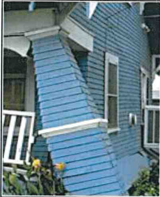
Figure 11. Earthquake Damaged Front Porch
