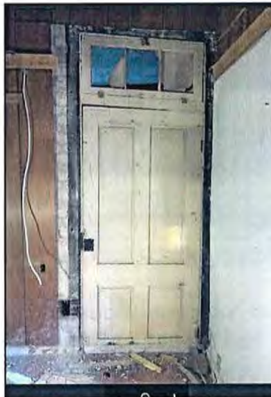
Original Door found Under by Modern Materials
