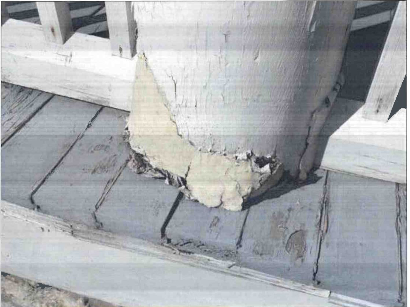
Photo 52 Previous repairs to the column bases are also failing.
