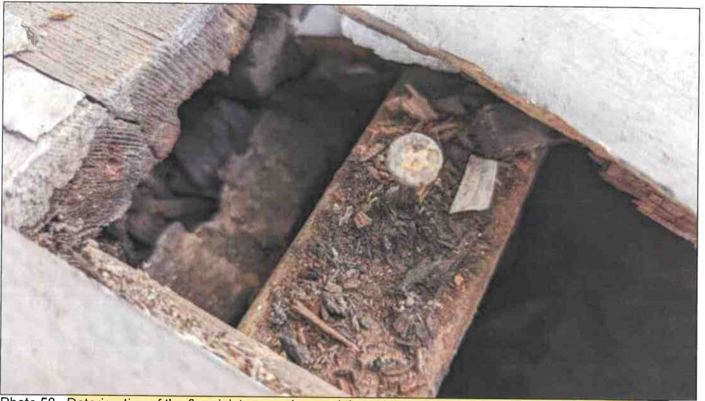
Photo 58 Deterioration of the floor joists was observed through the removal of some of the floorboards.
