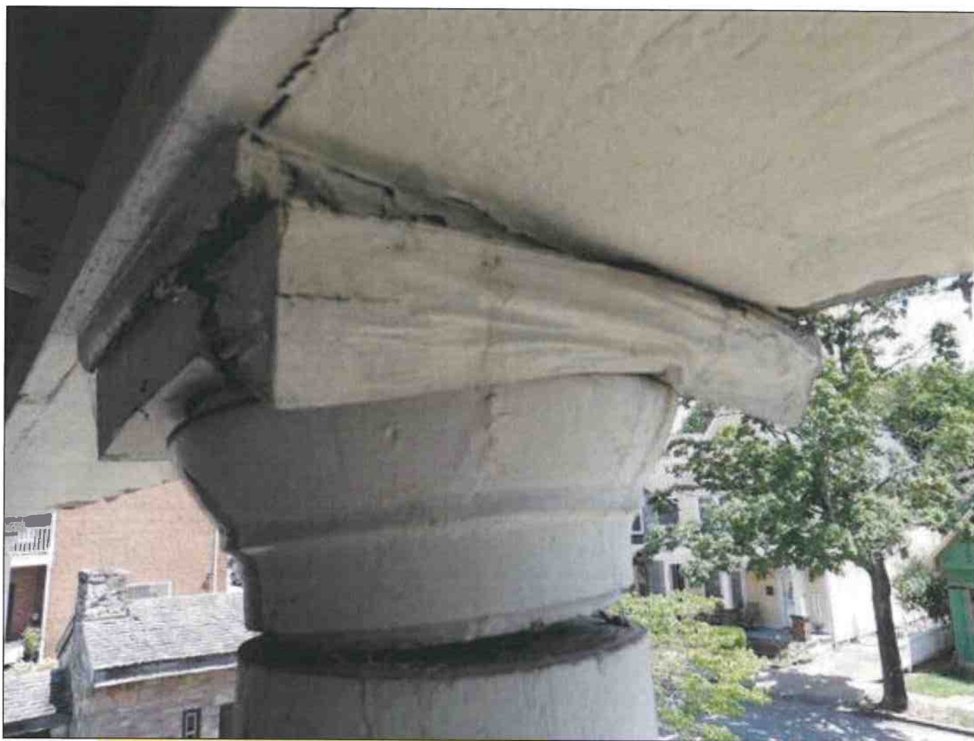
Photo 50 Deterioration was obvious within the column capitals.
