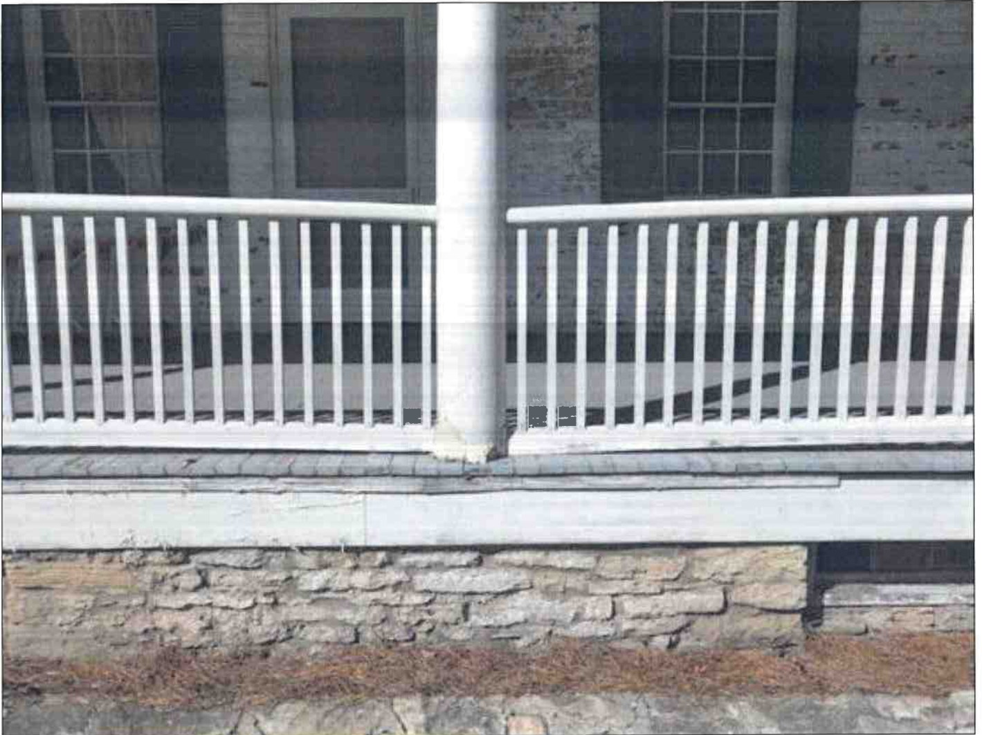
Photo 43 Displacement was obvious near the columns.
