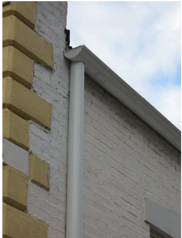
Gutters are recommended to be half-round design with round downspouts (510 E. Second Street).
