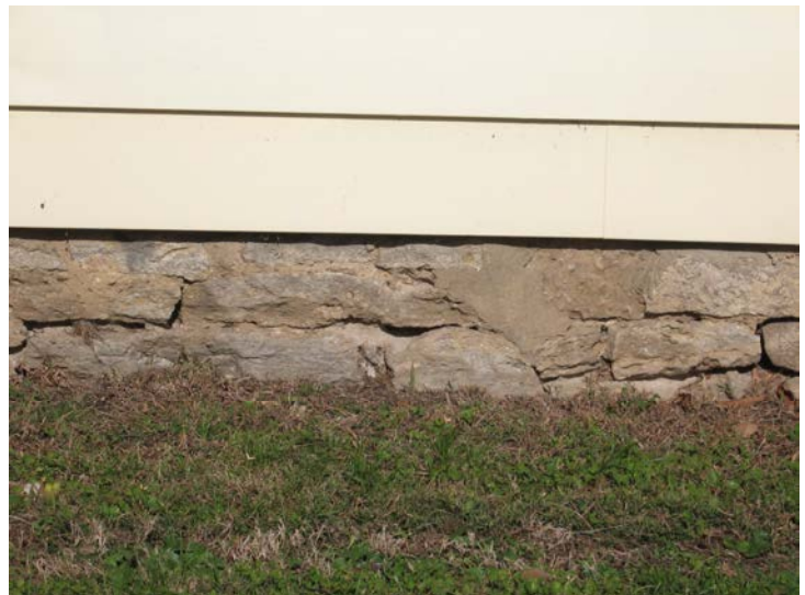
Stone foundation at 1002 W. Second Street.
