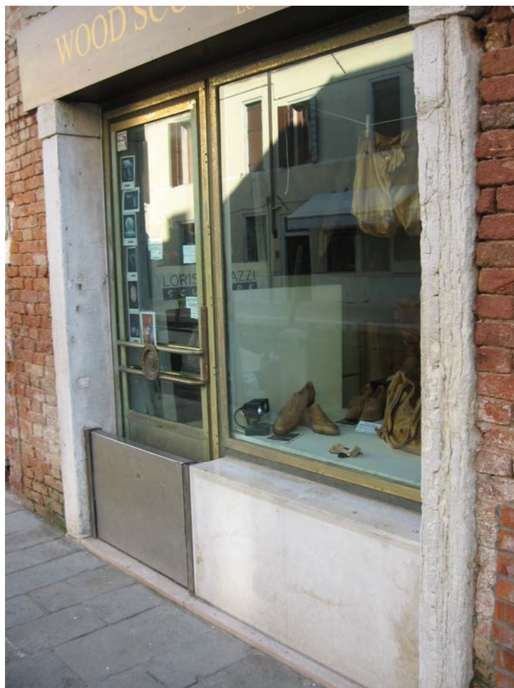
Dry floodproofing may include the installation of temporary flood panels at doorways and storefronts as shown above and below.
