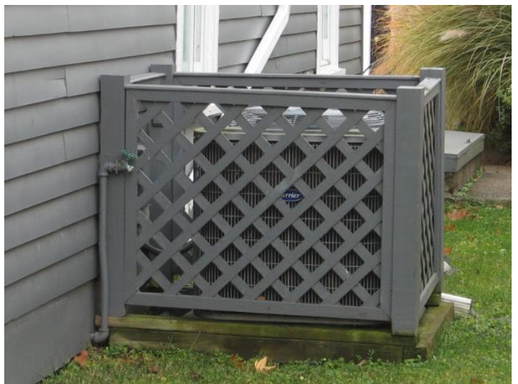
YES: This mechanical unit is appropriately screened by lattice panels (201 Walnut Street).
