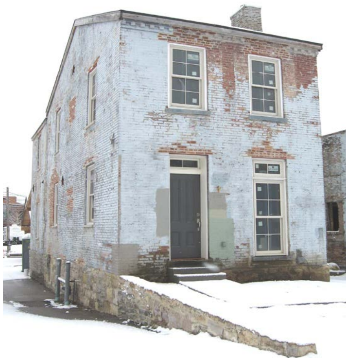
Rehabilitation projects may include the addition of a compatible door, appropriate replacement windows and the cleaning and painting of exterior masonry (613 Mulberry Street).
