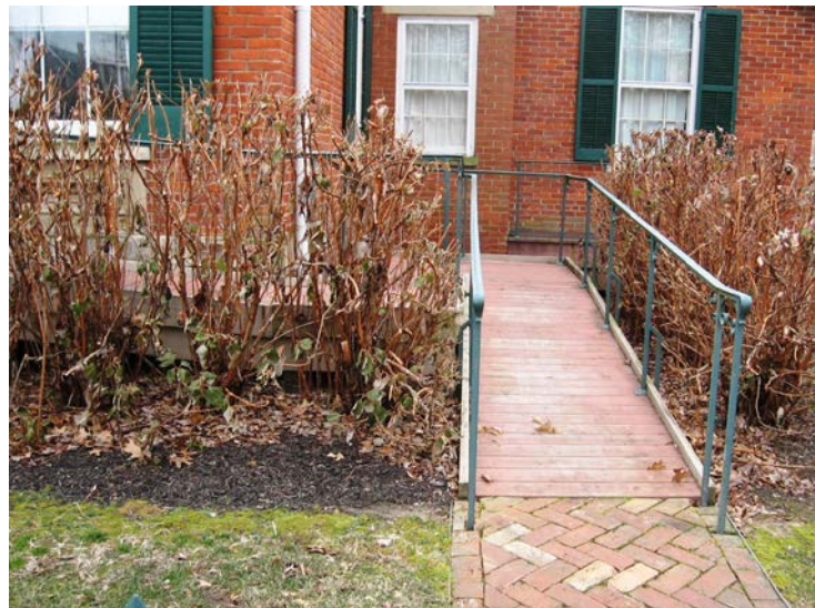
YES: At 301 W. Main Street is an ADA ramp with a simple metal handrail and screened by landscaping.
