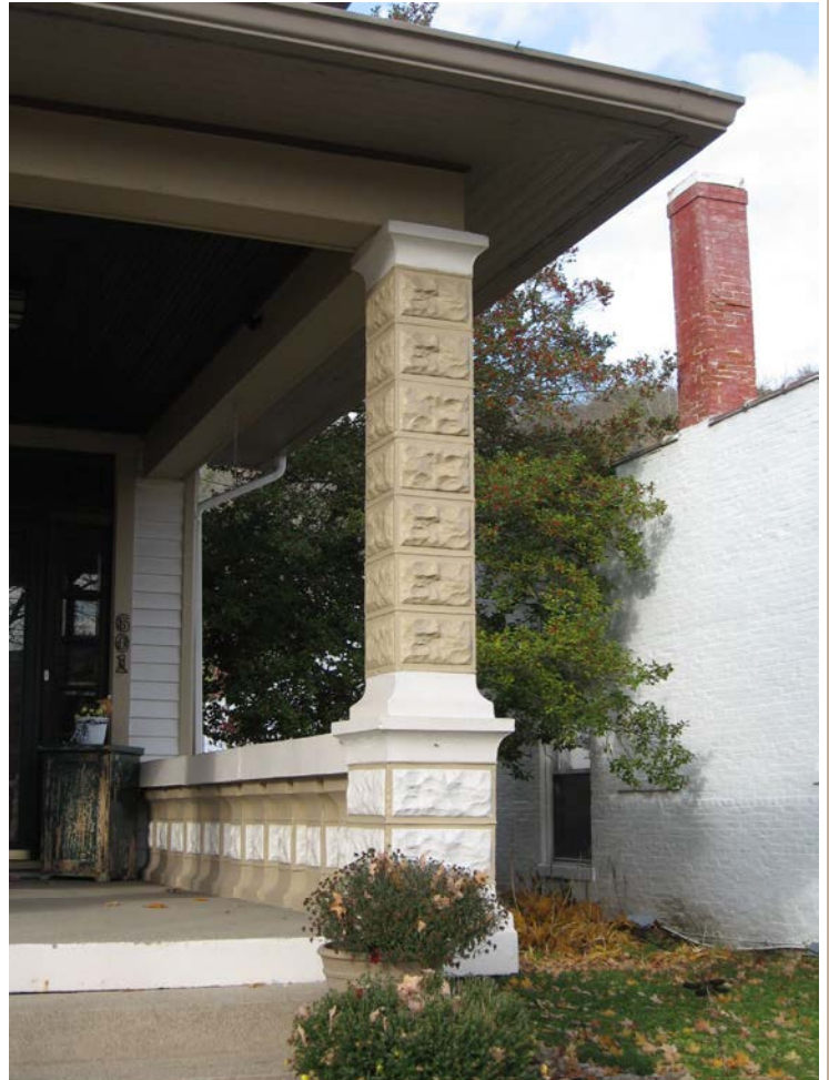
Rustic or rock-faced concrete block was used as a material for foundations and porch columns on some dwellings in the historic district (601 E. Main Street).
