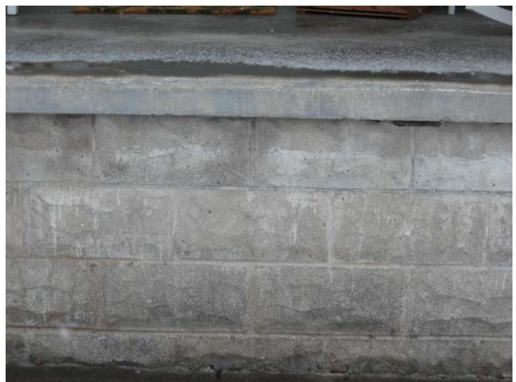
Rusticated (rock-faced) concrete block foundation at 209 Presbyterian Avenue.
