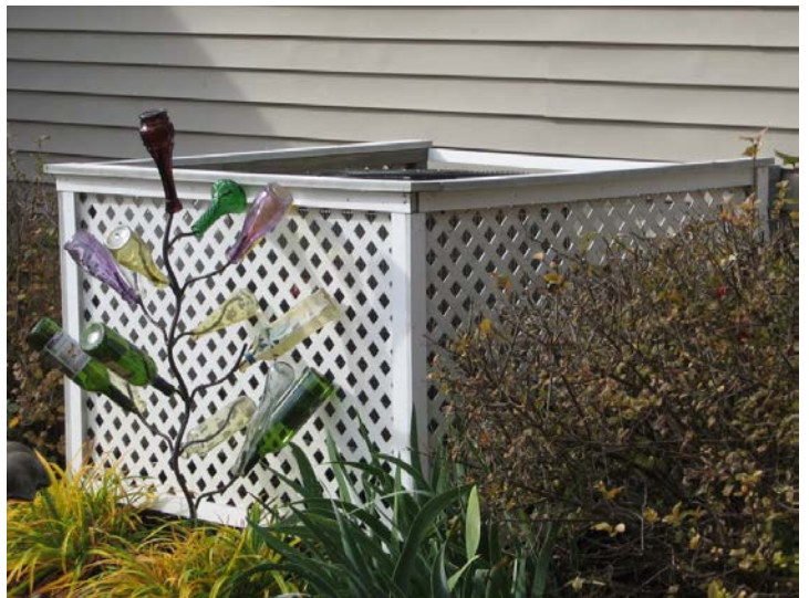
YES: Lattice and landscaping may be used to screen outside utilities on side and rear elevations (201 W. First Street).
