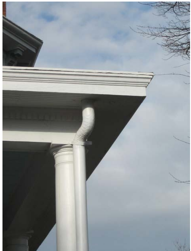
Preserve and maintain ca. 1900 box gutters like the ones added to the ca. 1860 home at 934 W. Main Street.
