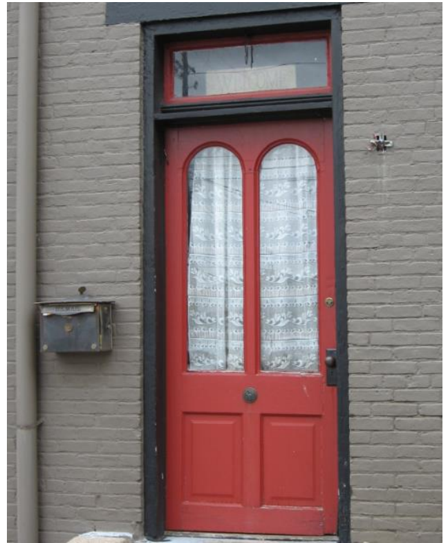
An entrance can be an appropriate place for a pronounced color contrast (317 Central Ave.).
