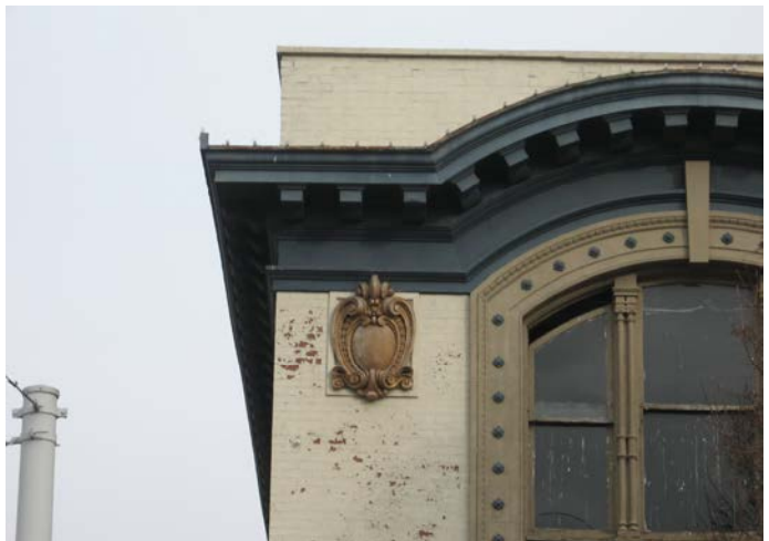
Decorative features of terra cotta and similar materials are also evident on some upper facades (101 E. Main
