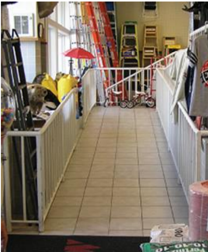
After entering the business, shoppers can either use an ADA compliant ramp (left) or go up the stairs to the new first floor level (right). The entrance area has been retrofitted with flood resistant materials including a tile floor and tile surfaces on the stairs.
