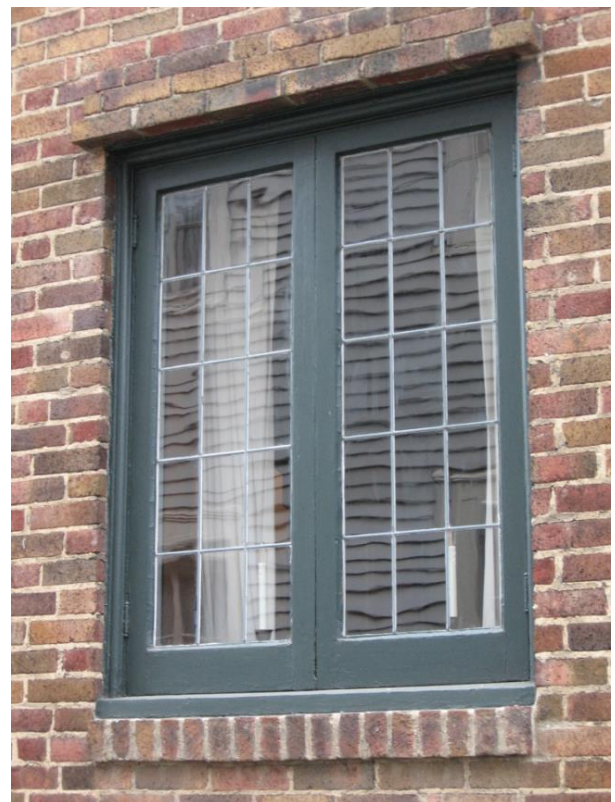
Casement windows are common features for early twentieth century Revival style dwellings (213 W. Second Street).
