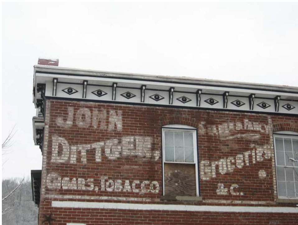
“Ghost signs” which remain on commercial buildings should be preserved and maintained (624 West Street).
