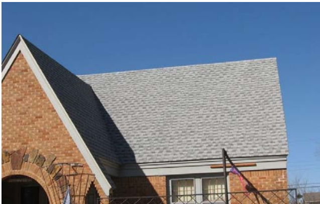
Reflective roof shingles may be appropriate for some dwellings. These assist in lowering cooling costs in warmer months.
