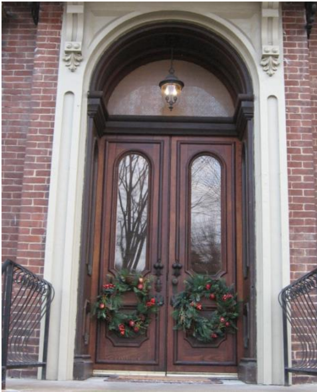
Italianate style doors were often designed with arched glass lights as at 512 E. Main Street.
