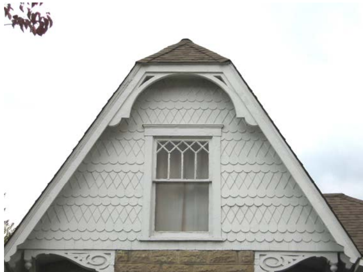
Many dwellings feature decorative wood shingles in gables or as exterior wall materials (523 Jefferson Street).
