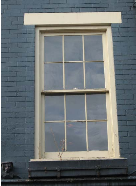
Six-over-six wood sash, 207 W. Main Street.
