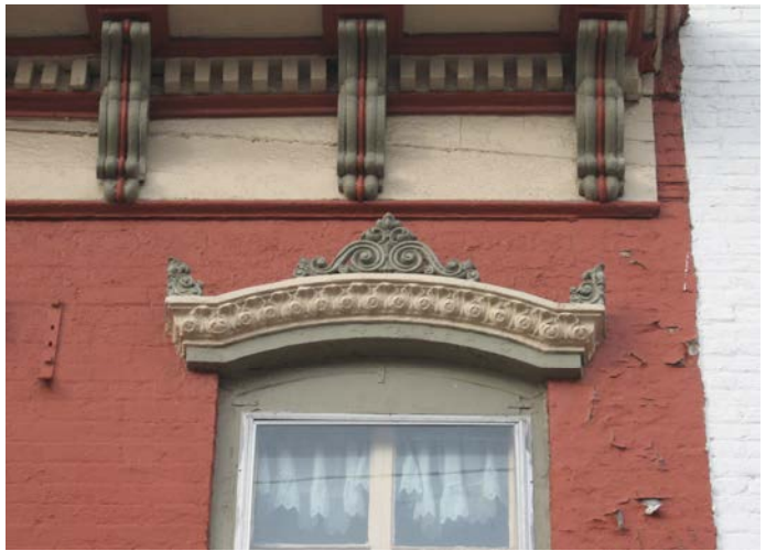
Architectural details can include cast iron hood moldings over windows and sheet metal cornices at rooflines (321 Mulberry Street has cast iron hood moldings over its windows).
