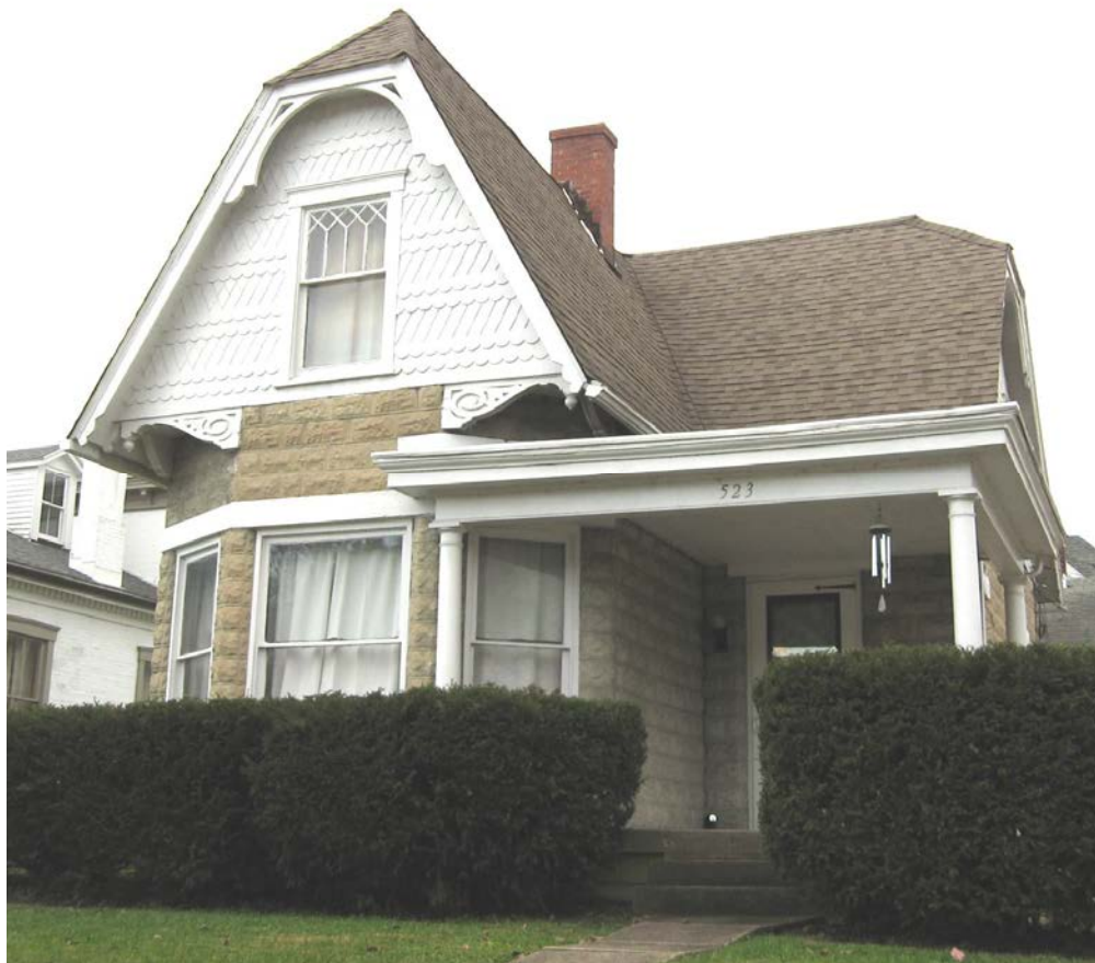
Rustic or rock-faced concrete block was used as an exterior wall material on a number of dwellings built in the early 1900s (523 Jefferson Street).
