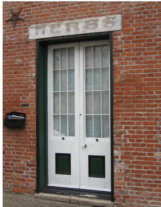
Original glass and wood double doors at 318 Mulberry Street.
