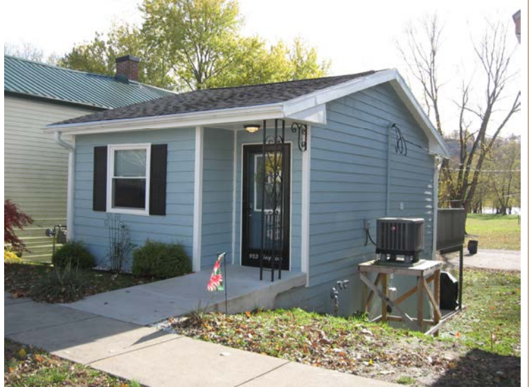
The property at 923 W. First Street has an elevated mechanical unit on a wood platform.
