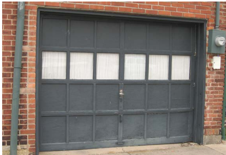
YES: Replacement garage doors should be based on historic designs such as the roll-up door of wood and glass at 302 Jefferson Street.
