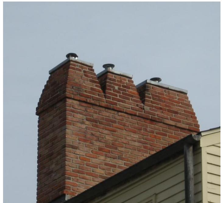
Preserve and maintain decorative chimneys and chimney caps such as this distinctive triplet set at 217 W. Second Street.
