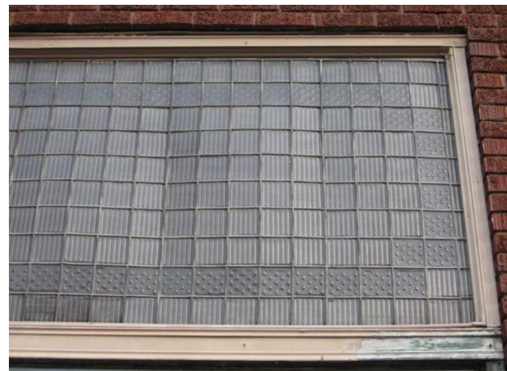
Do not permanently cover or conceal storefront transoms like this Luxfer glass example (125 E. Main Street). Retractable canvas awnings may be added to storefronts and might cover storefront transoms while closed.
