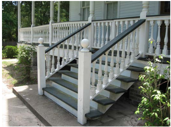
YES: Rebuilt stairs should match the dwelling's original porch design and detailing.
