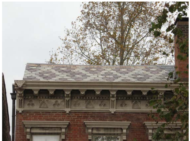
Slate roofs are often distinguishing features of a dwelling (507 Broadway Street).
