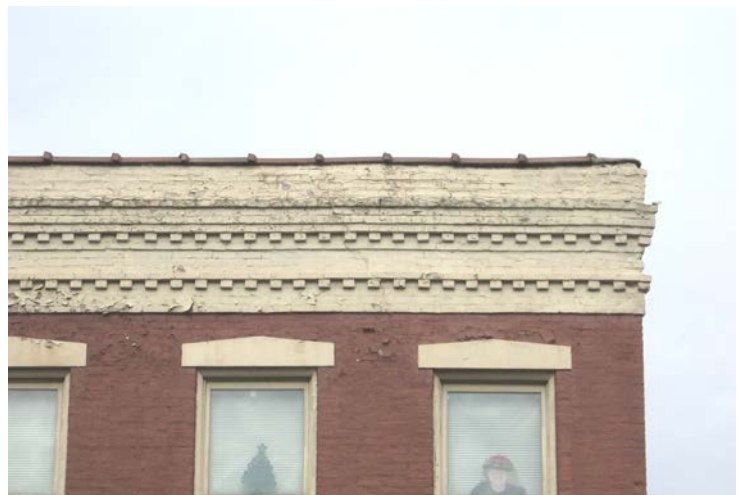
Several commercial buildings also display cornices of corbelled brick as at 100 W. Main Street.
