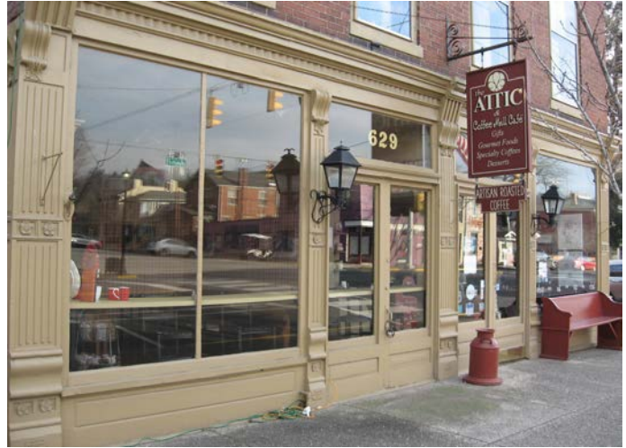
The mid-nineteenth century building at 629 W. Main Street was remodeled at a later time with a cast-iron storefront.
