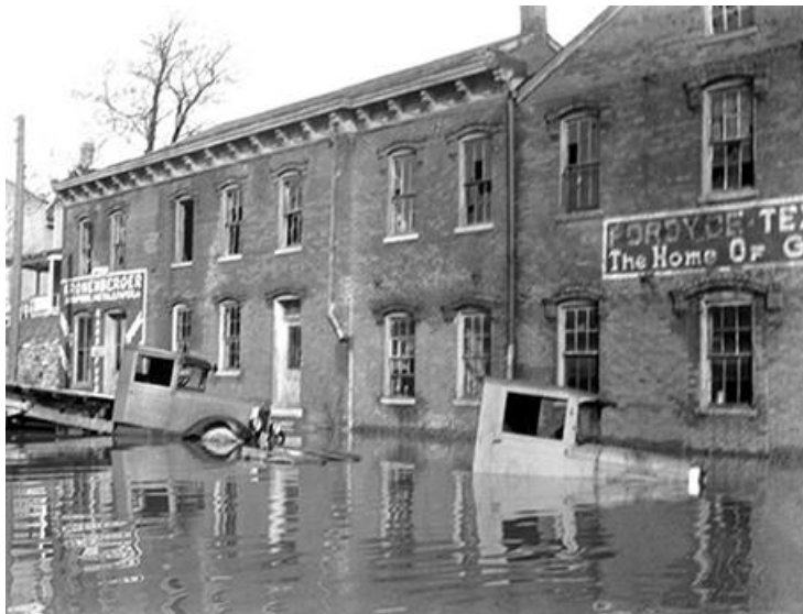
The 1937 flood devastated many of the industries along the river. This view shows the Fordyce Textile Mill at 200-202 Jefferson Street. This building still stands at this location. (Photo courtesy of the Madison-Jefferson County Public Library).
