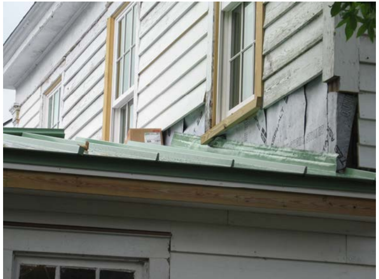
YES —This roof is appropriate since it has traditional standing seam profiles and spacing.
