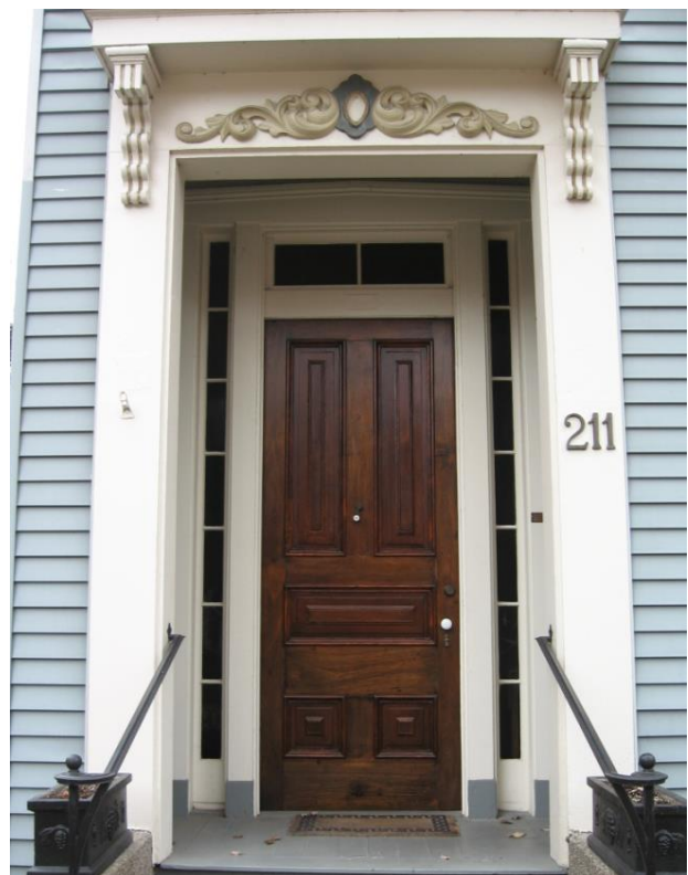
Preserve and maintain all entrance elements such as sidelights, transom, and door surrounds (211 W. Second Street).
