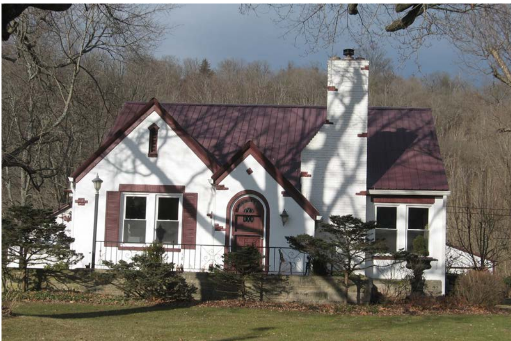
Chimneys are often character-defining features of particular styles such as this prominent chimney on the Tudor Revival dwelling at 1218 W. Main Street.
