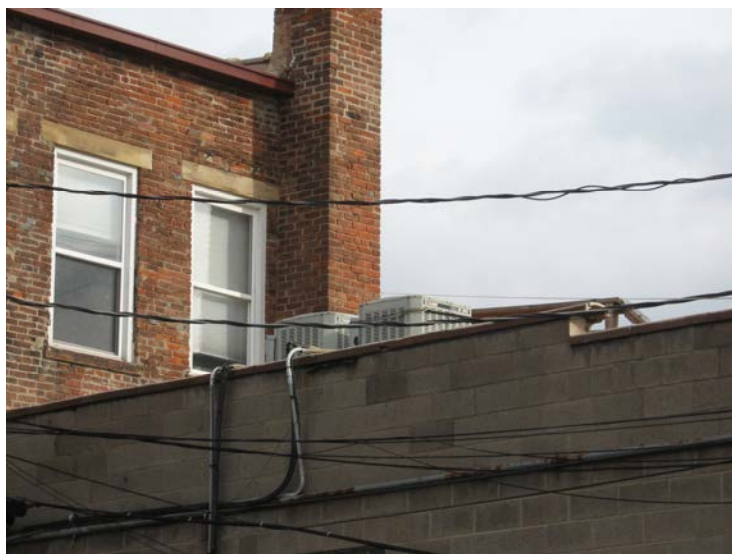
YES: On commercial buildings, mechanical units may be sited at rear elevations or on roofs not readily visible from the public right-of-way as at 110 E. Main Street.
