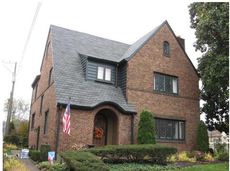
The dwelling at 213 W. Second Street has an arched entrance bay and original casement windows.
