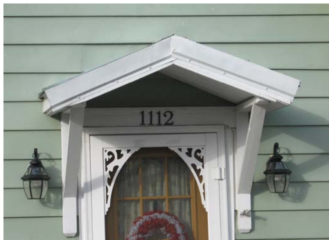
Wood canopies over doorways are common features in the historic district especially on early 20th-century homes (1112 W. Main Street).
