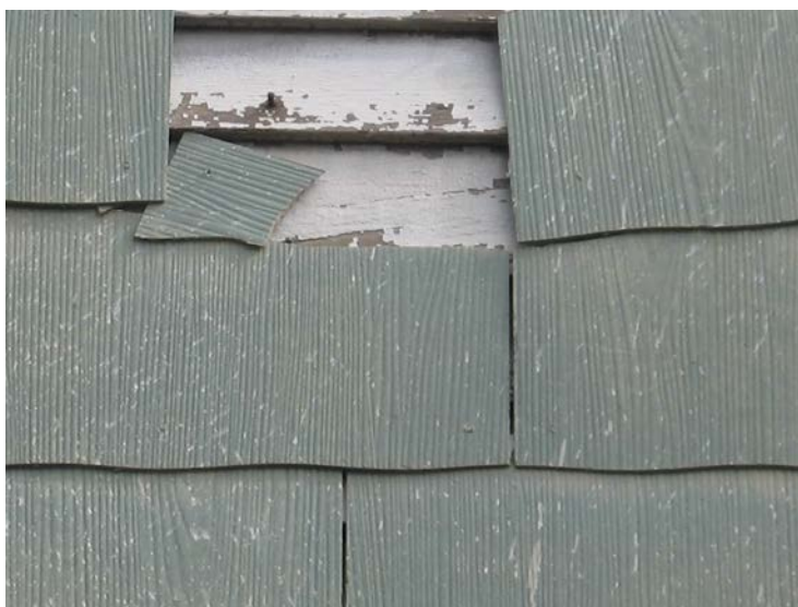
Removal of asbestos shingles and restoration of the original wood siding is encouraged.
