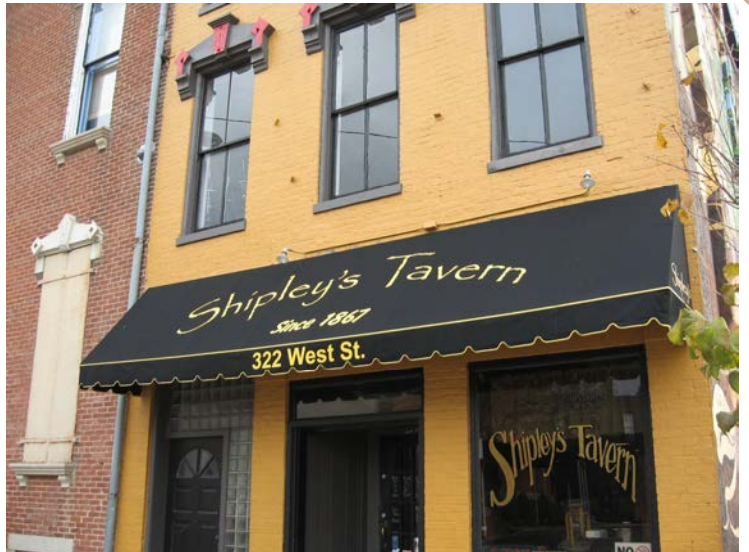
Awnings are traditional sign locations (322 West Street).
