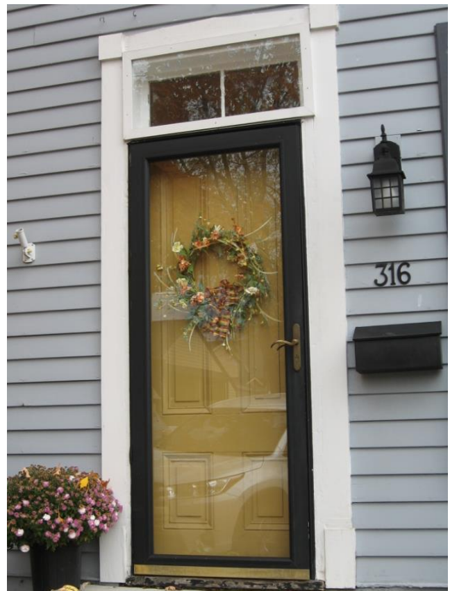
YES -Full-view storm doors are appropriate which allow for the visibility of the historic door behind it (316 Mill Street).
