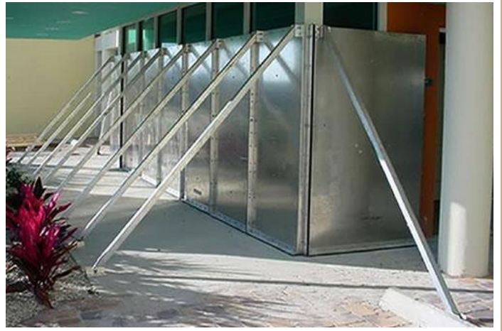
Temporary flood panels are now widely available to protect downtown commercial buildings. When high water events are anticipated these can be erected to minimize flood damage.
