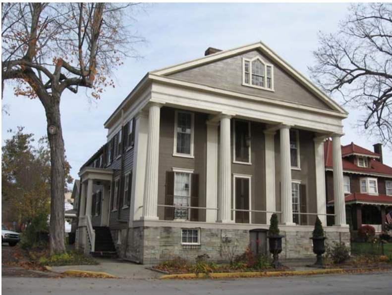
The dwelling at 302 Elm Street, built in 1838, features a two-story Doric portico on a raised basement.
