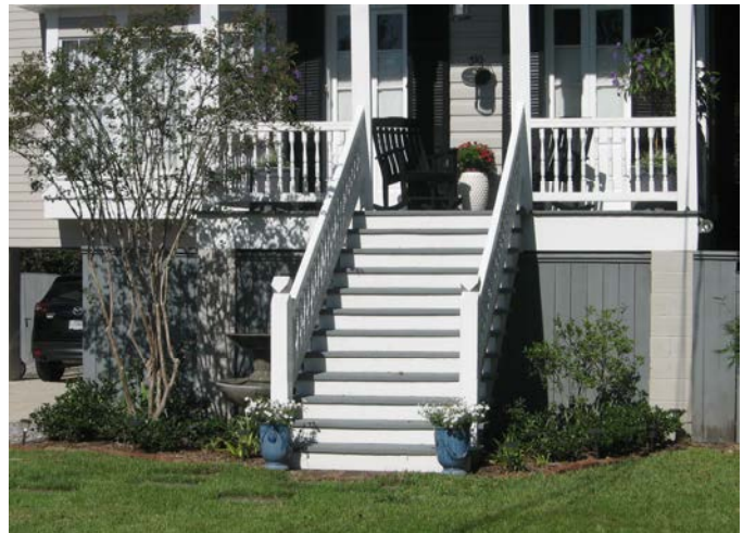
YES: This low elevation project has a new wood stair which complements the dwelling's style and design.
