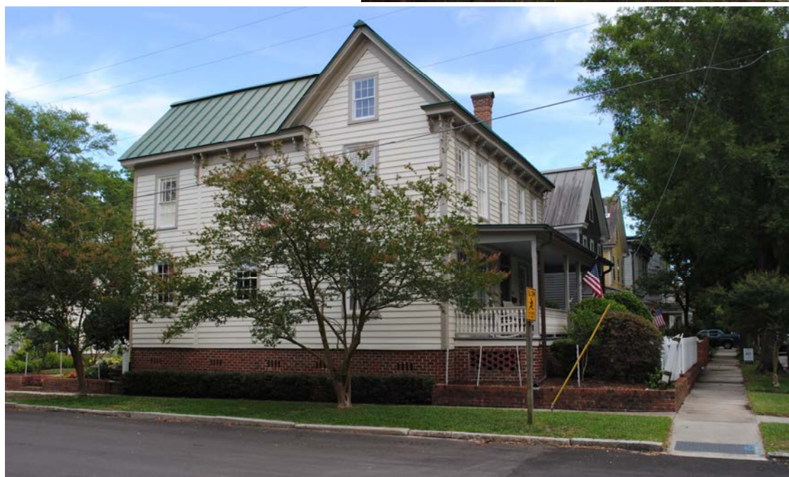
YES: The screening of this low elevation increase project includes a brick wall and landscaping to mitigate the increased height of the foundation.
