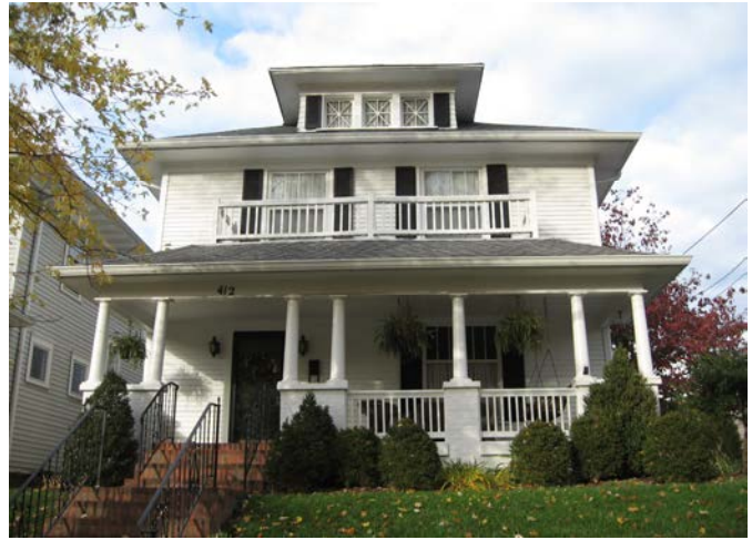
At 412 W. First Street is an example of the American Foursquare style with a full-width porch with Tuscan columns and a hipped dormer at the roofline.
