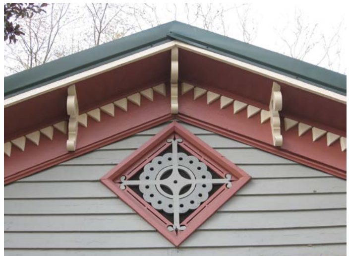
Architectural details may also include eave brackets and a decorative attic window (1057 W. Main Street).
