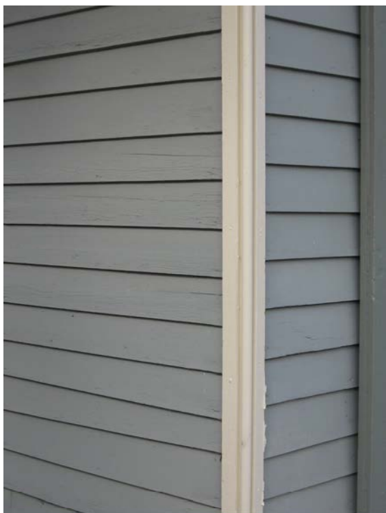
In addition to the wood siding, preserve and maintain original corner boards, fascia boards and other wood features (1057 W. Main Street).
