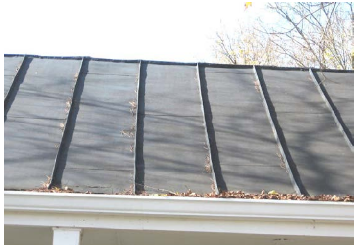
Metal standing-seam roofs from the nineteenth and early twentieth centuries should be preserved and maintained (902 W. First Street).
