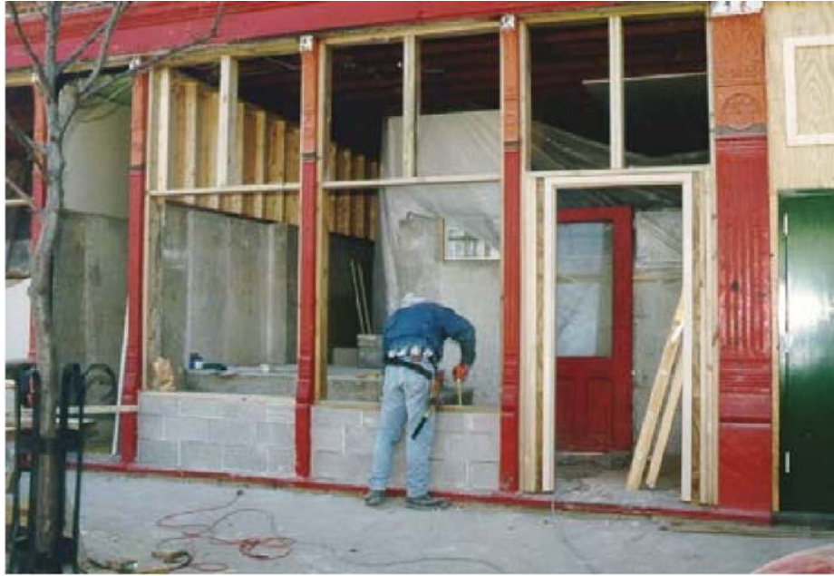
Another strategy for floodproofing commercial buildings is to harden the storefront and raise the interior first floor level. In this approach the frame storefront bulkheads are replaced with concrete and a parged surface (above). (Photos courtesy of FEMA, Darlington, Wisconsin).
