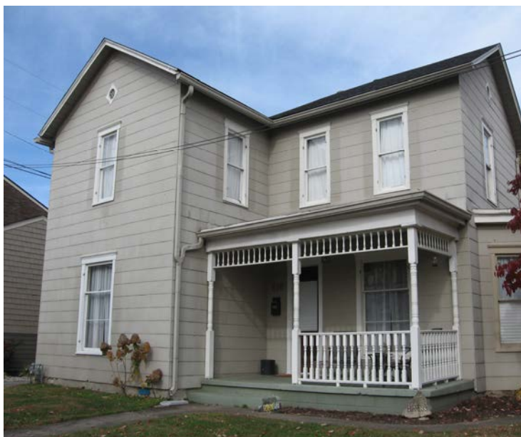
A number of dwellings in the historic district had the original wood siding covered with asbestos shingles in the mid-twentieth century (410 W. Second Street).
