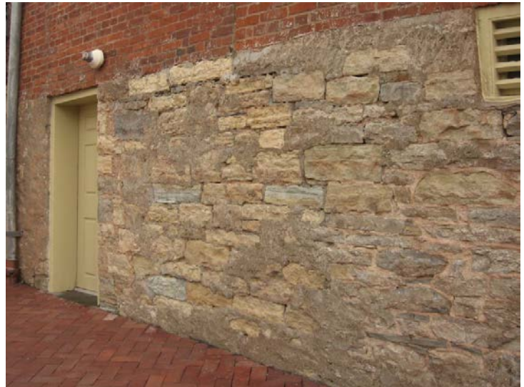
Stone foundation at 217 W. Second Street.
