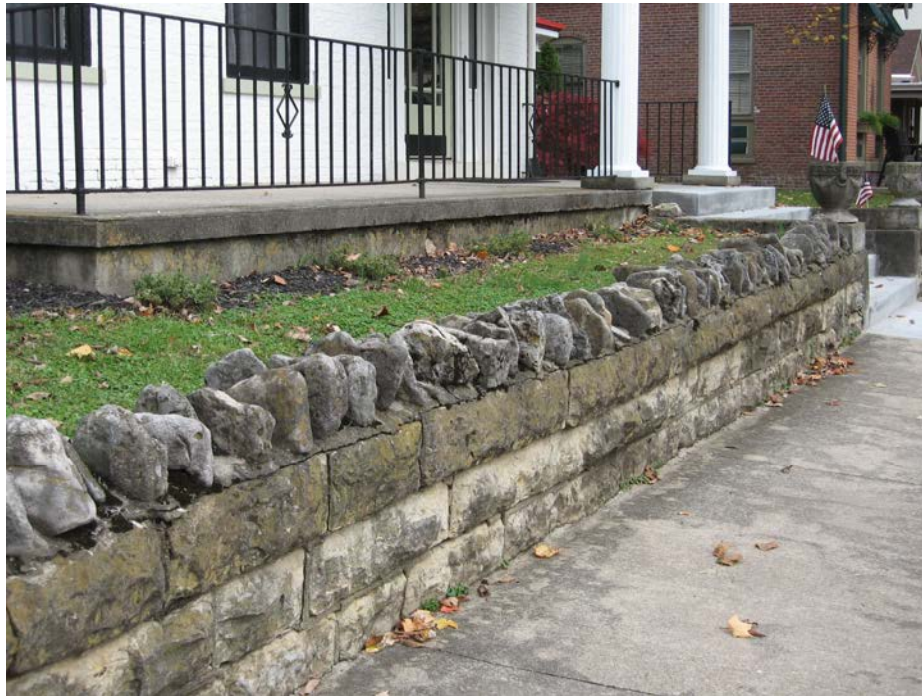
Front yard retaining walls of stone or rusticated concrete block should be preserved and maintained (624 W. Second Street).
