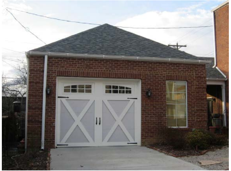
YES: The new garage at 315 Poplar Street is appropriately scaled, and its garage door is based on traditional designs.
