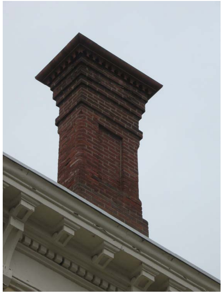
The chimney at 402 W. Main Street was built with details reflecting its overall Italianate design.
